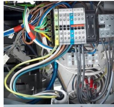
Connect the mains connection cable to the terminals PE to N according to the connection scheme. Observe the connection scheme fixed at the bulkhead of the electric installation compartment.
